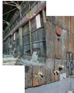
Materiality: Site Photos
